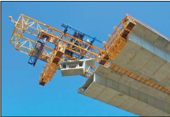
A segment is swung into position at the cantilever tip.
