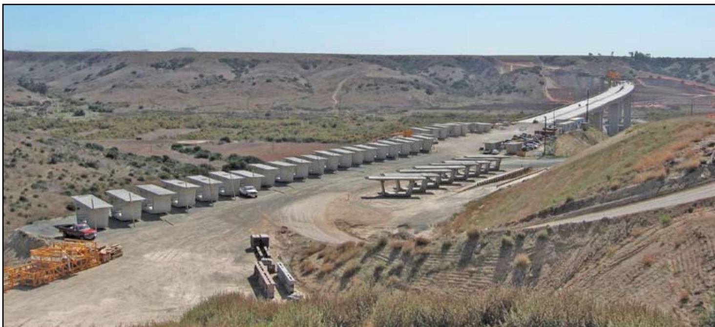
Segments wait in storage behind the completed spans.
